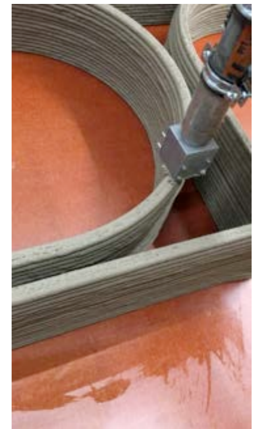
3D concrete printing
