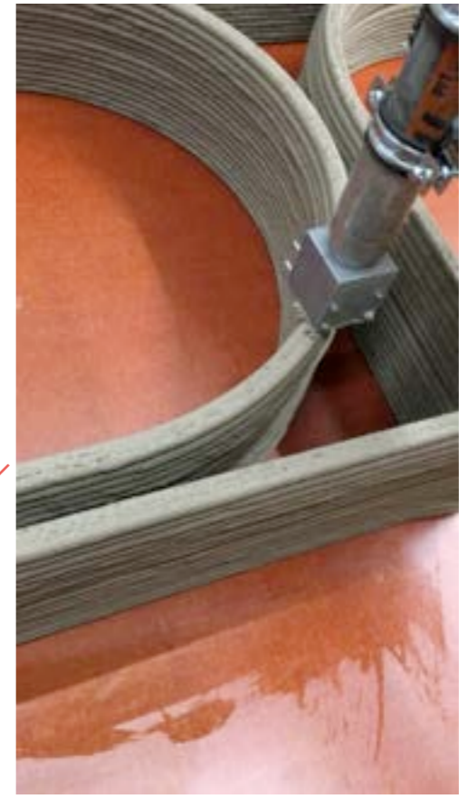
3D Concrete Printing
